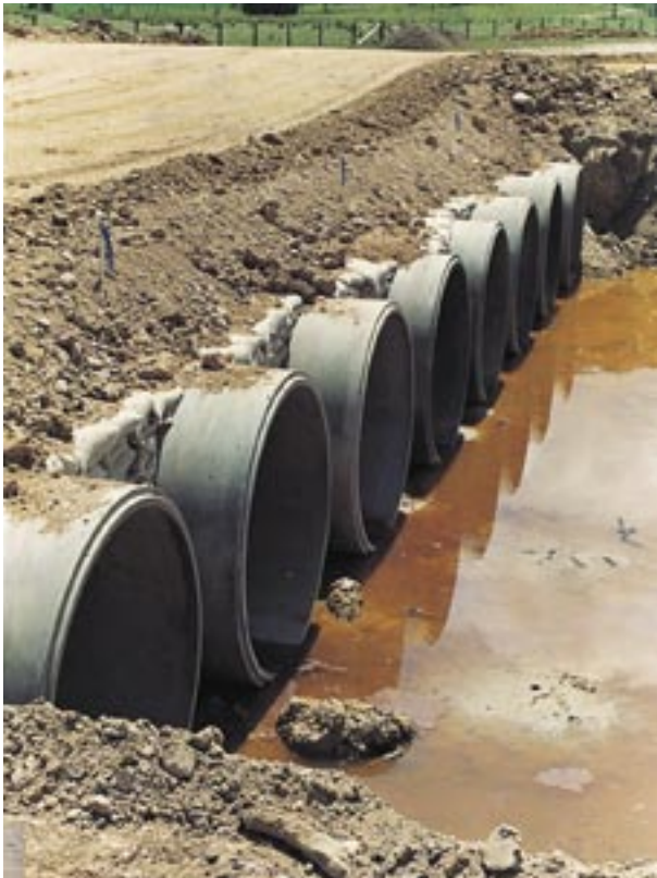
A typical multi-channel culvert during construction.
