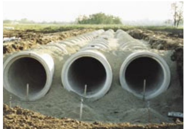
Multiple 1350 diameter Rubber Ring Joint stormwater pipes - Rocklea Markets Brisbane.
