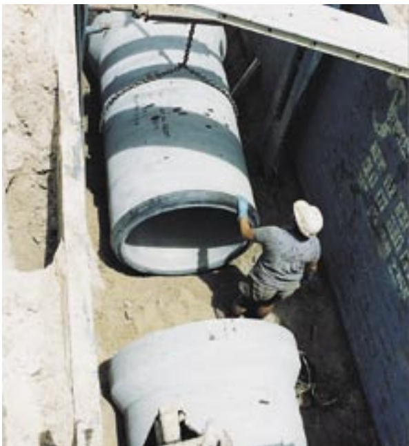
Jointing of large diameter sewerage pipes at Oxley Creek Brisbane.
