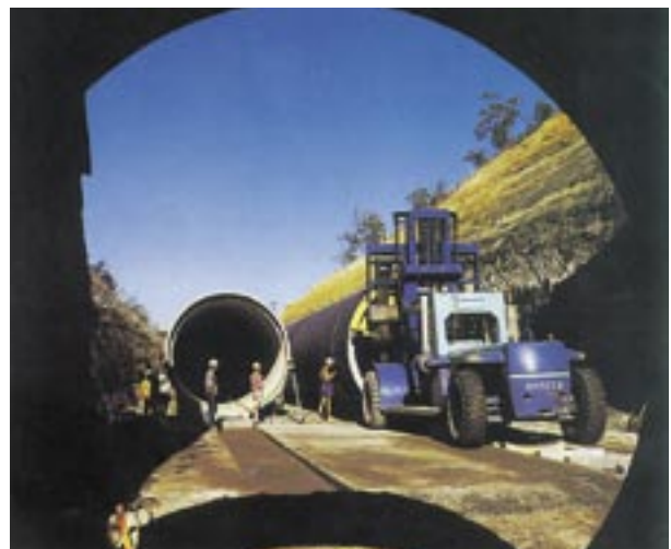
3600mm diameter pipes being installed at Prospect Dam - NSW.
