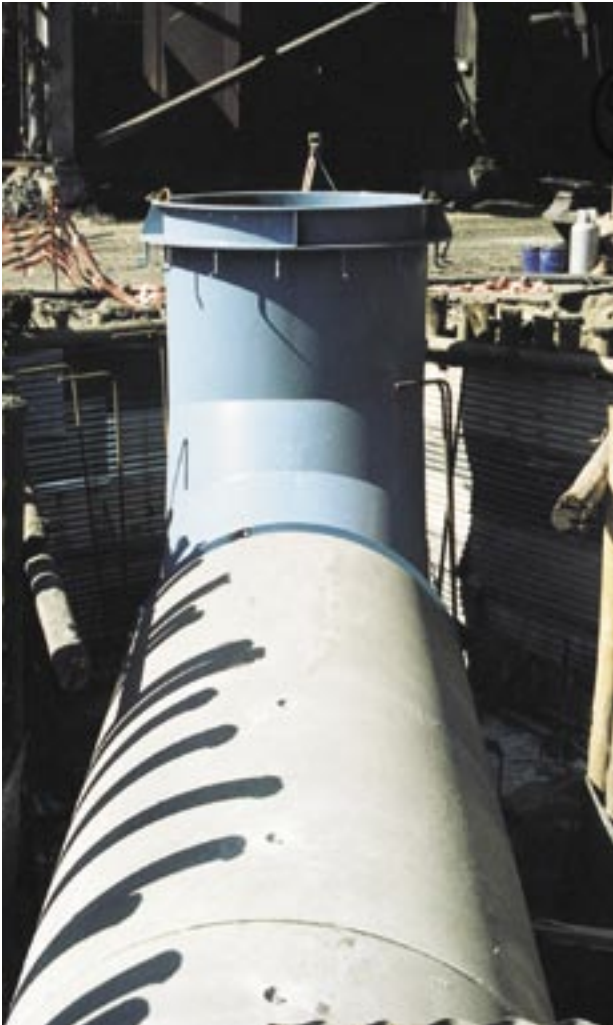
Mild steel adaptor for 2100mm diameter skid ring joint pipe.
