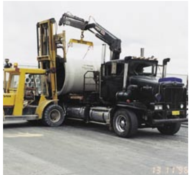
Concrete pipe being loaded onto truck for delivery to site.
