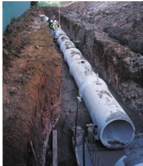
Bedding prepared, pipes laid ready to receive back fill.
