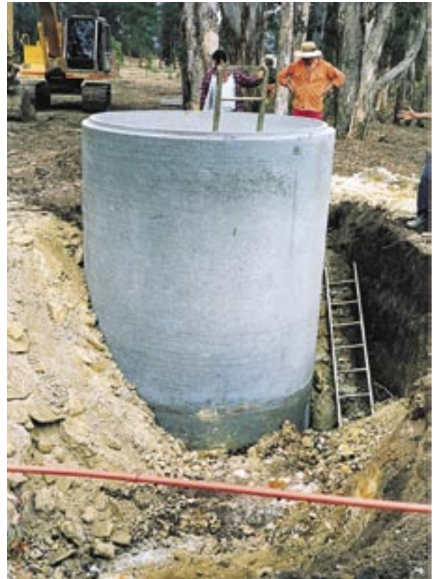
A precast pump station.
