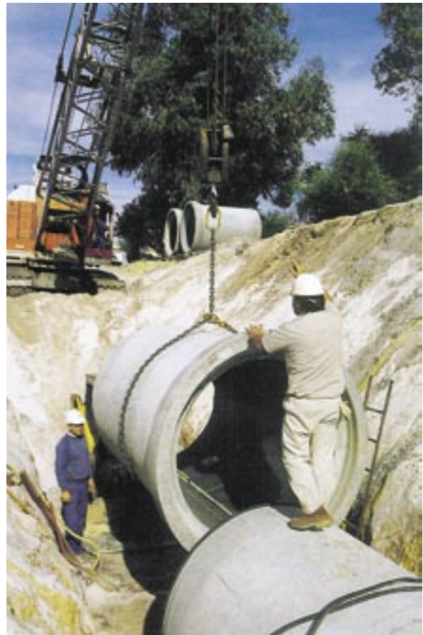
Sewerage pipe (Plastiline™) during installation.
