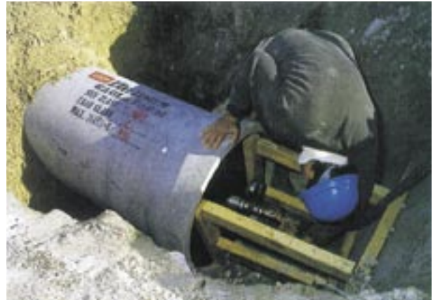
Field testing of pipes - Brisbane.
