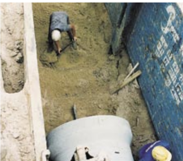
Preparing the bedding to accommodate the socket.
