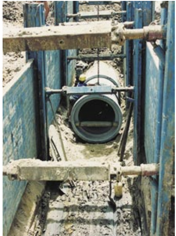
Installing sewer pipes, note trench shoring equipment (Oxley Creek - Brisbane).
