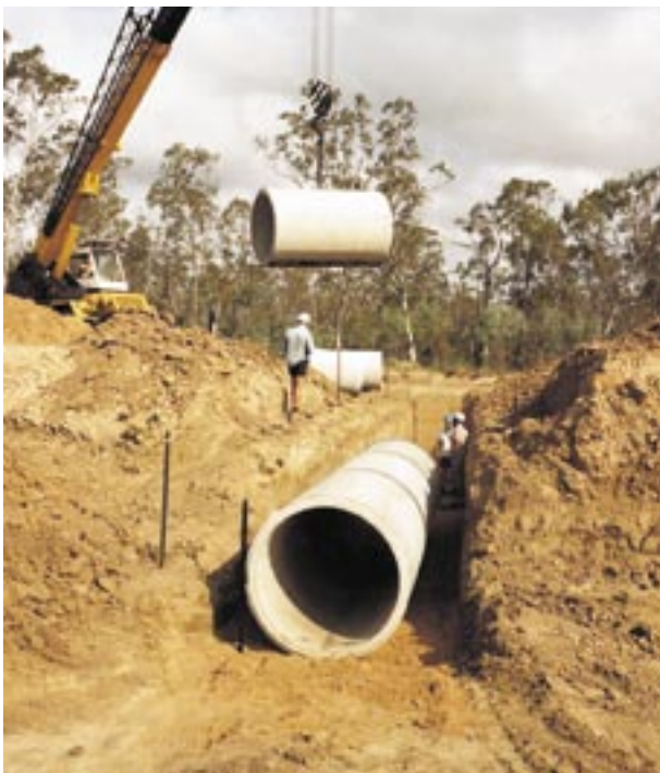
A trench installation for a rural culvert.
