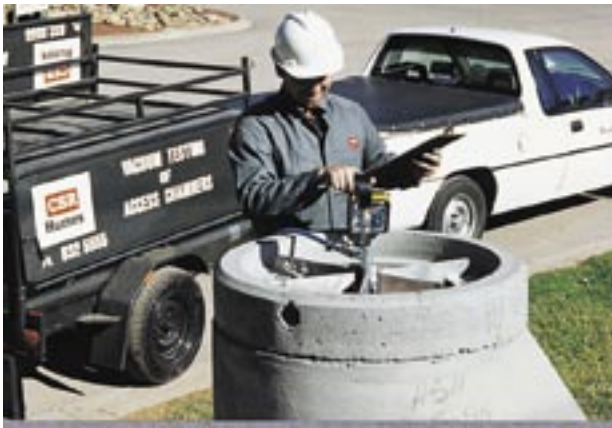
Vacuum testing of Access Chamber.
