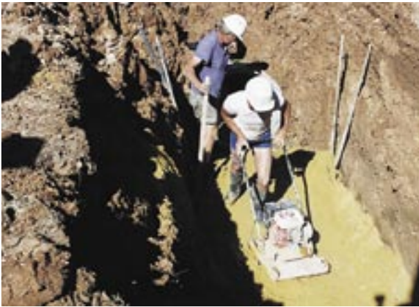
Compacting of fill material is a critical part of the installation
