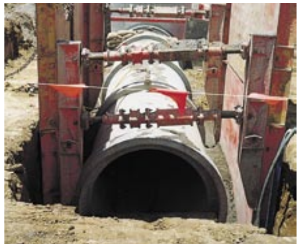
Large diameter Rubber Ring Joint Pipe installation at Goolwa - S.A.
