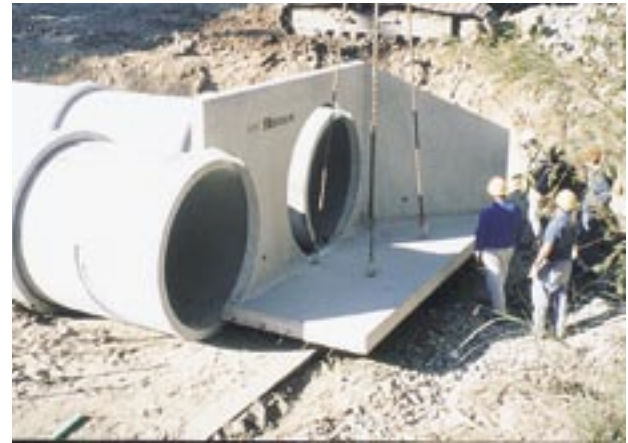
Precast concrete Headwalls for Rubber Ring Joint Pipes.
