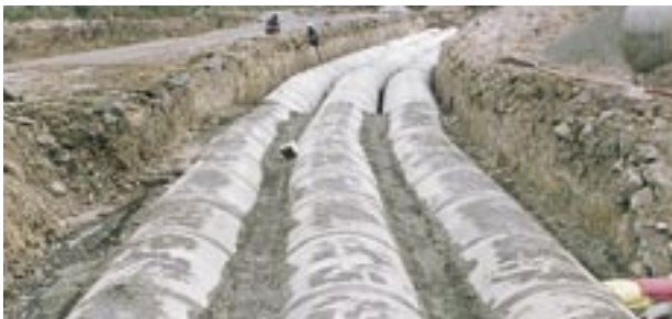
Multiple Barrel Splay Pipes (EB Joint).
