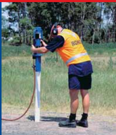
PNEUMATIC INSTALLATION
